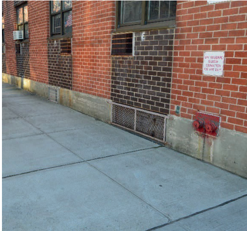
a. Ventilation openings near sidewalk level
