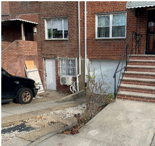
c. Driveway sloping down to converted basement
