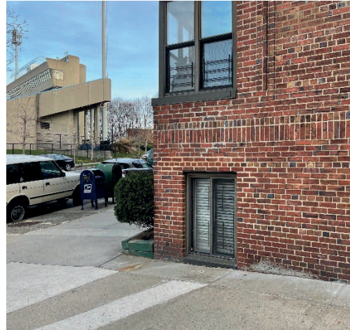
b. Basement window sill near sidewalk level
