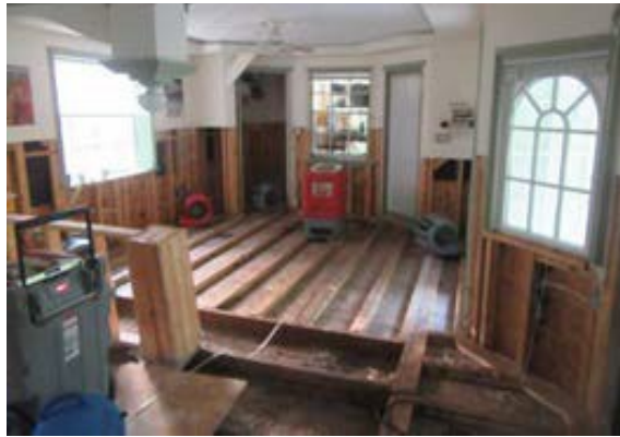
Figure 64: Sleeper System Installed Over a Concrete
