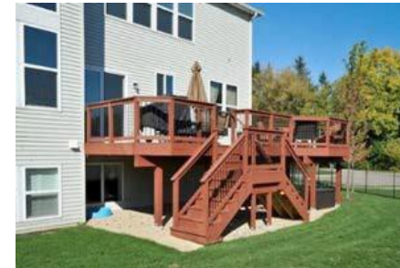
Figure 21: Deck with Double Staircase
