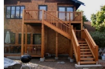
Figure 38: Deck with Single Set of Stairs
