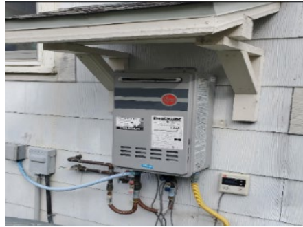
Figure 63: Wall-mounted Tankless Water Heater
