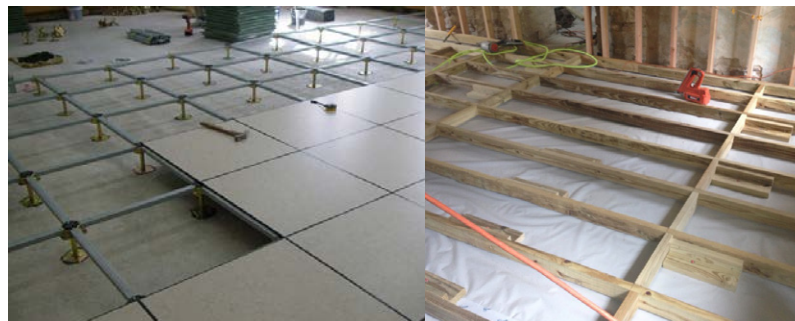
◀ False/raised floor (left); sleeper system installed over concrete (right)
