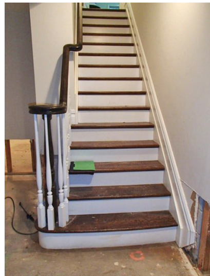
▲ Finished stairs are not covered.
