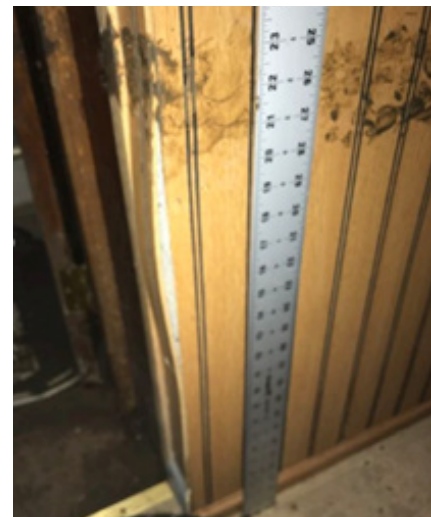
▲ Example of a questionable photograph: no flood debris, would not support a recommendation of damage by or from flood.
