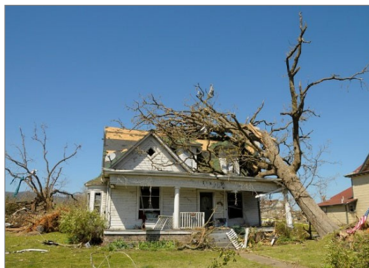
A home in Arkansas is damaged by a fallen tree.
