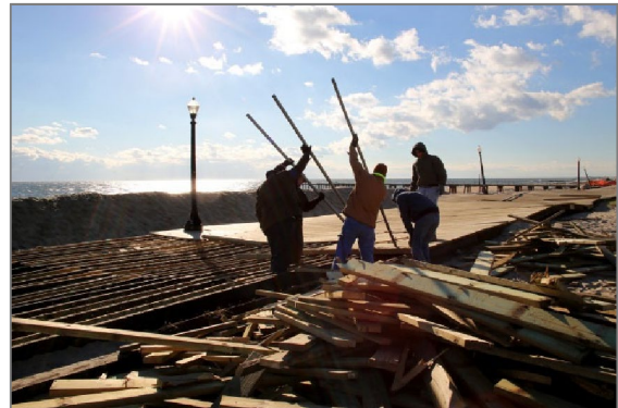
The Calvary Chapel Relief volunteers, an organization, works tirelessly to remove damaged boards from the Asbury Park boardwalk after Hurricane Sandy.
