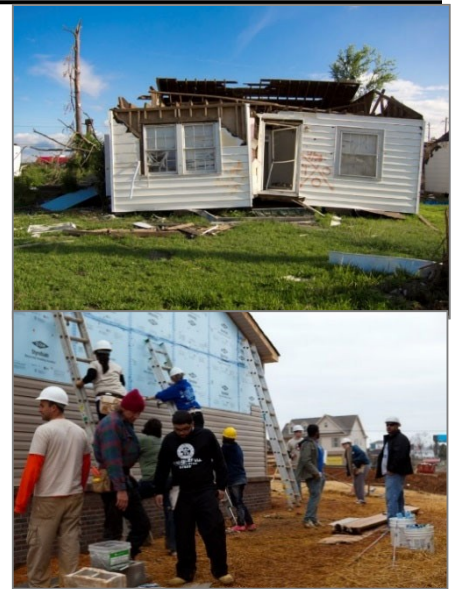
Above: A disaster-destroyed home. Below: Volunteers repair a home.
