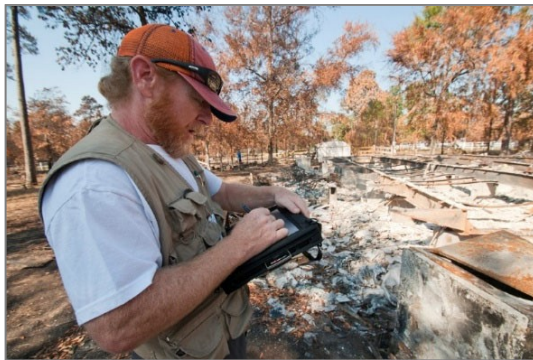
A FEMA inspector verifies wildfire damage at a severely impacted home site in Texas.
