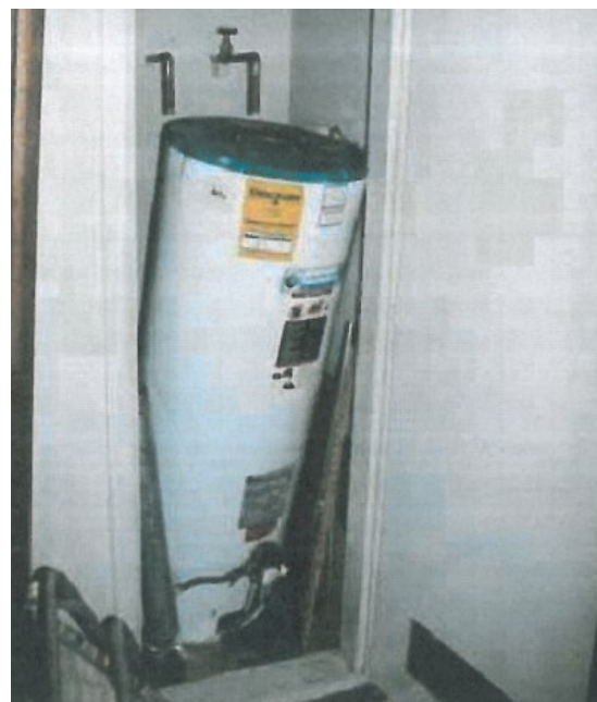
Photo of water heater failure in 1994 Northridge Earthquake.
