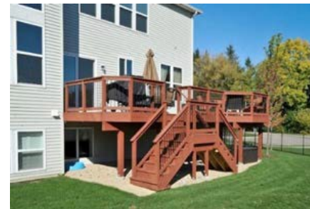
Figure 18. Deck with Double Staircase
