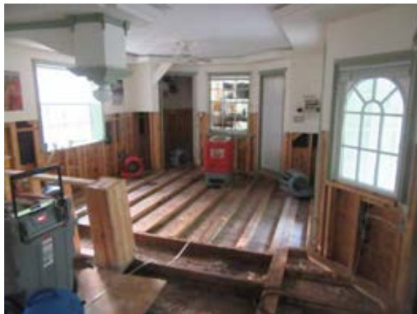
Figure 31. Sleeper System Installed Over a Concrete
